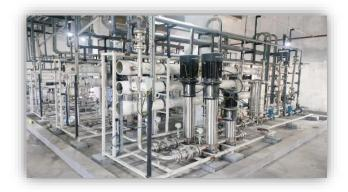
Building on these systems, MRF has installed 400 KLD and 300 KLD wastewater recycling plants at two of its plants to convert treated wastewater into RO-quality process water. Steam condensate recovery has also been integrated into operations, where process condensate is reused in cooling tower and AHU applications at one of our plants, reducing the need for fresh make-up water.
